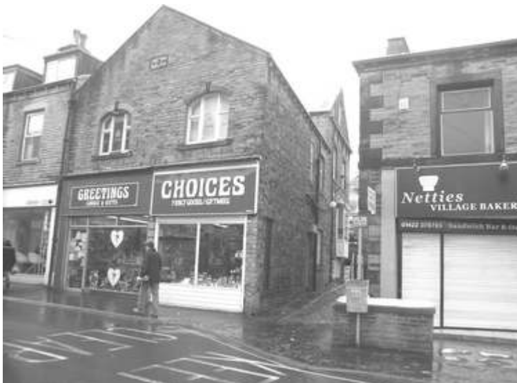
Under the Choices sign is the shop at 58 Southgate, Elland, as it is today. The building has been modified slightly at some point, but is essentially the same
